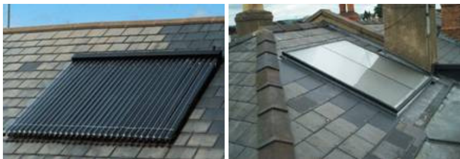
Two common types of solar collector: evacuated tubes (left) and flat plates (right)
