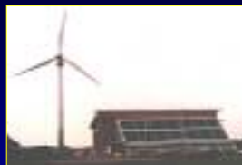
1.5 MW wind turbine at Ecotech Centre
