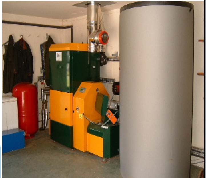
60 kW KWB Chip Boiler, with accumulator tank. Photo courtesy of Midlands Wood Fuel
