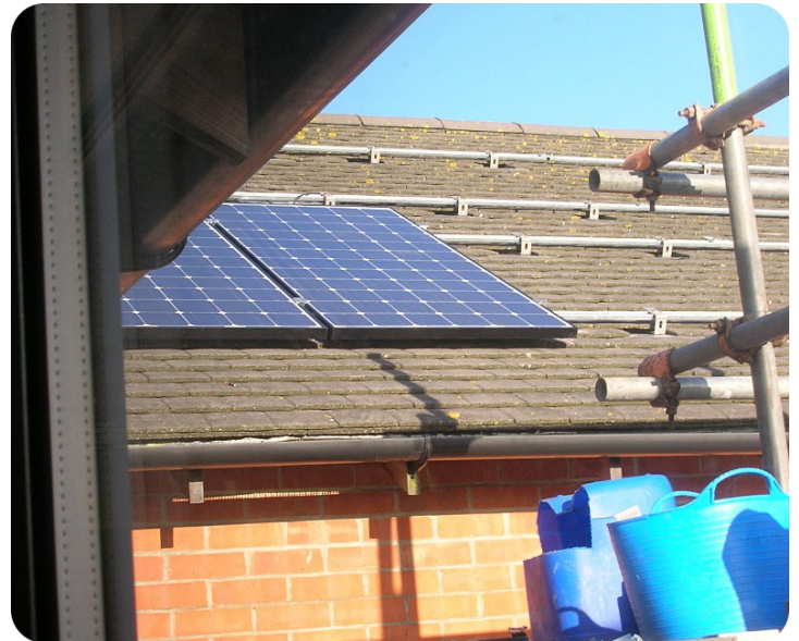
The unistrut frame systems that support the PV arrays only required the removal of a few roof tiles, and were installed in just two working days
