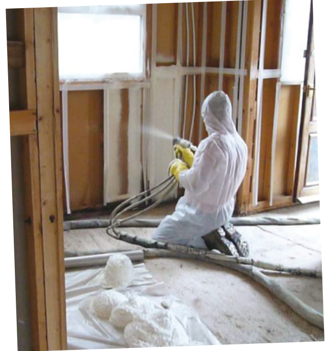
Spraying foam insulation into timber frame walls
