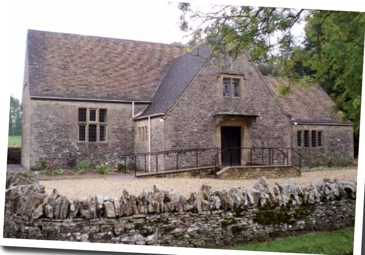
Miserden Village Hall showing the type of challenge that many village halls face with solid stone walls, single glazed windows and located within a conservation area
