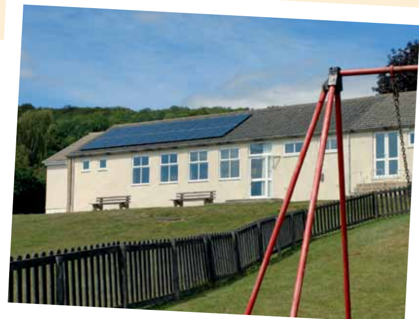
Newly-refurbished Randwick Village Hall with efficient double glazed windows and solar photovoltaic system on display
