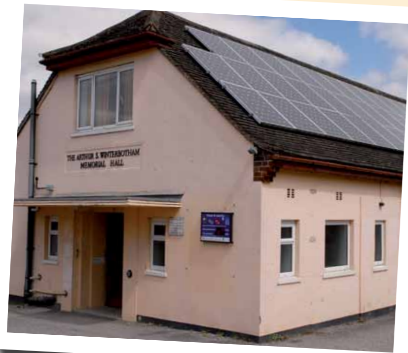
The Memorial Hall with 12kW photovoltaic system and information panel as viewed from Cam High Street
