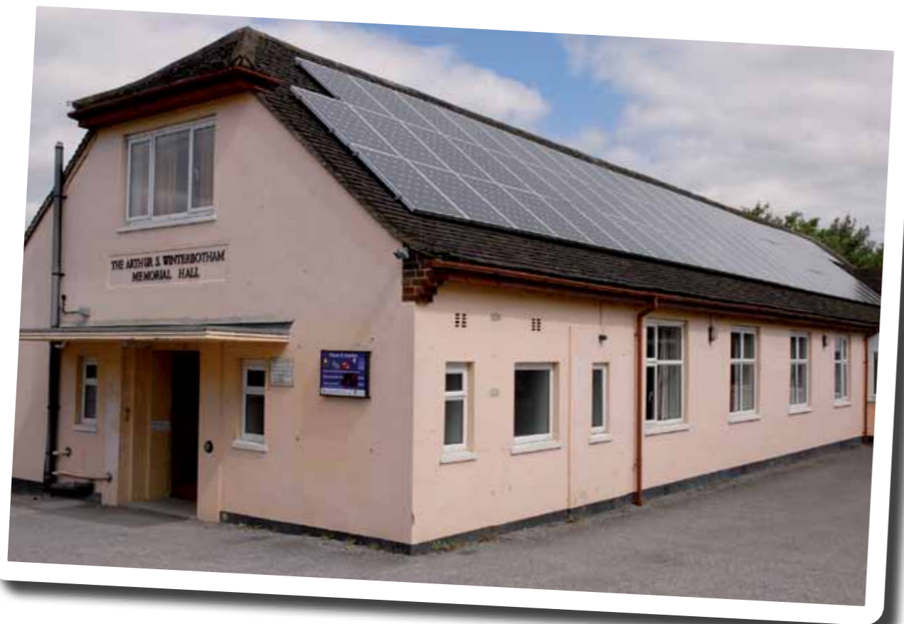
The 12kW solar photovoltaic system installed at Cam Memorial Hall
